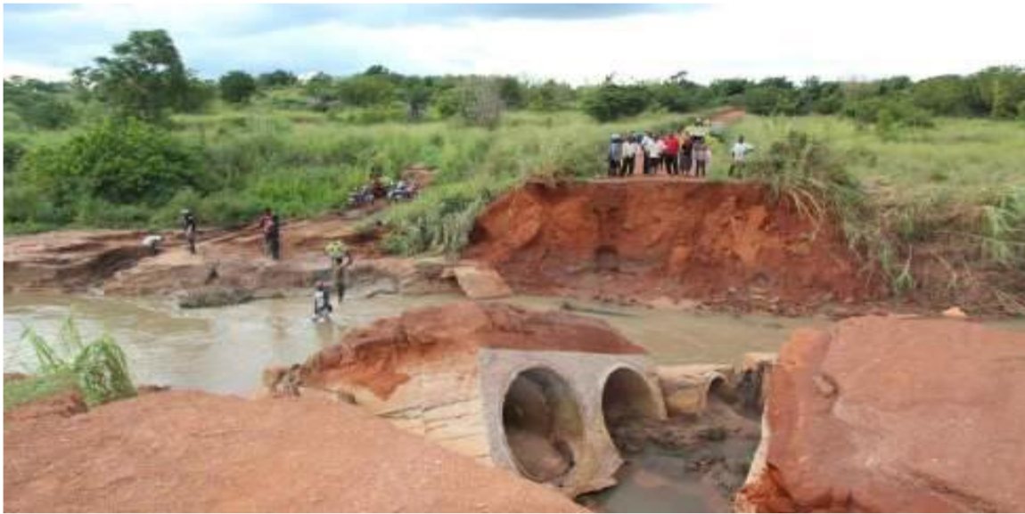
Photo 1 A culvert over River Bontire near the town of Abrewapong leading to the EcoPlanet Bamboo LLC's plantation in North Bandai Hills Forest Reserve, Juaso Forest District, Ashanti Region, washed away by heavy rains.
